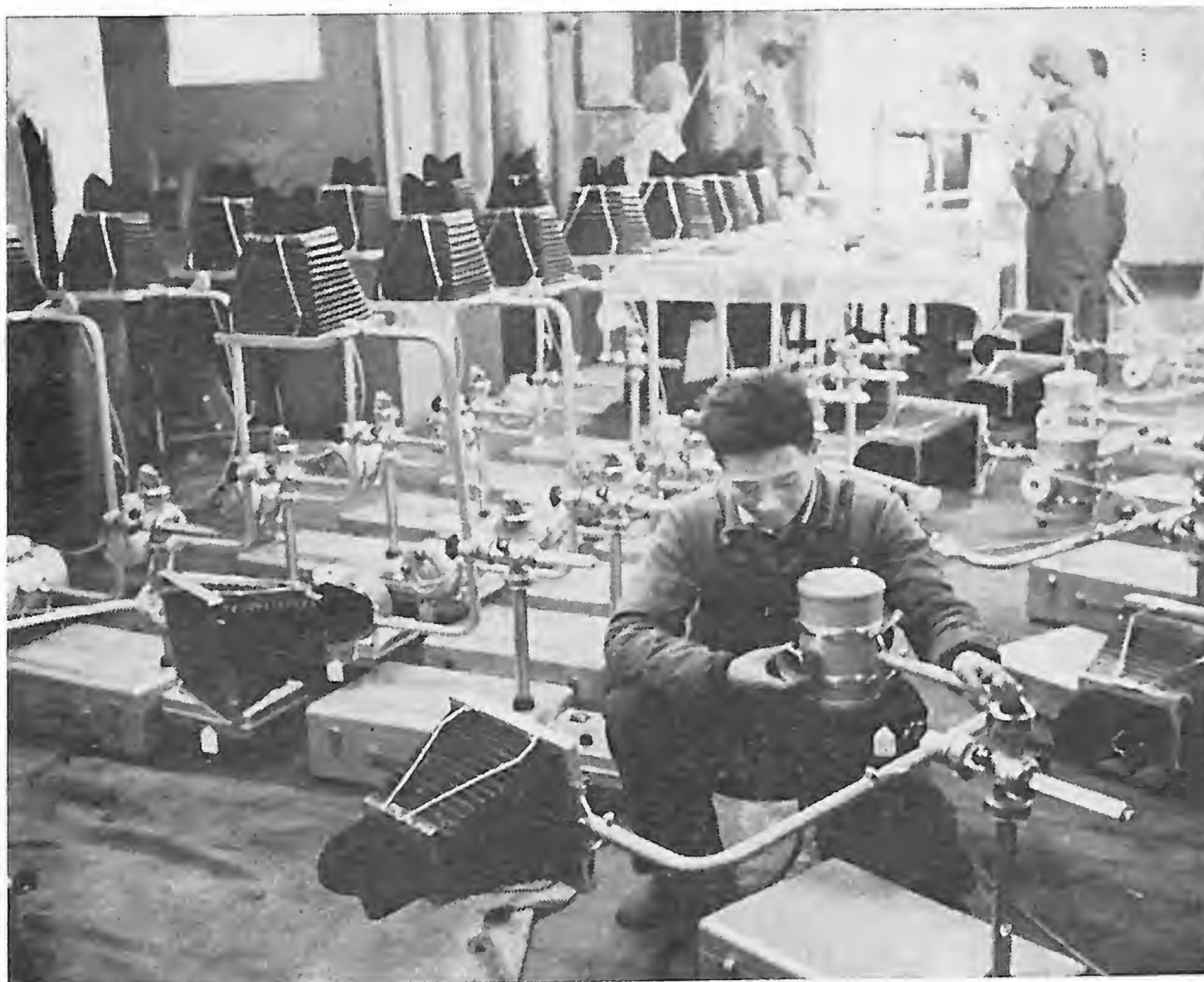
Portable diagnostic X-ray machines being assembled by workers at the Shanghai Medical Apparatus Plant.
